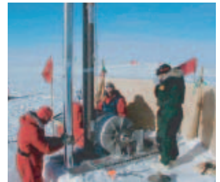
GSN seismic station QSPA at South Pole, Antarctica. The construction of this station required the drilling of boreholes in the ice to the depth of nearly 1000 feet. Photo shows the NSF contracted drillers operating the ice core drill at the QSPA site (~5 miles from the South Pole).
